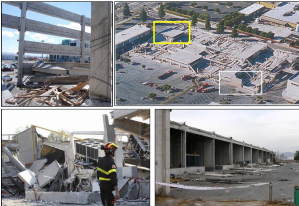
Figure 8: Precast concrete failures in past earthquakes.
