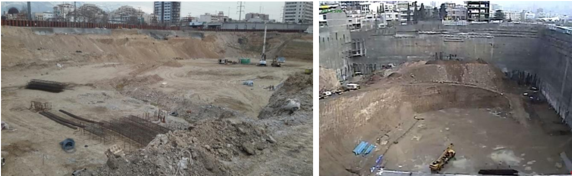
Figure 11: Examples of excavations in Tehran, Iran for high rise building construction.
