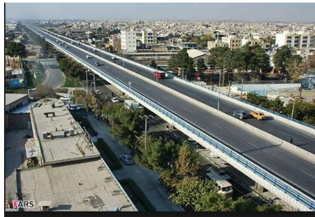
Figure 10: Double deck freeway in Isfahan, Iran.
